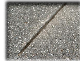
Floor Cutting : 8 x 12mm
